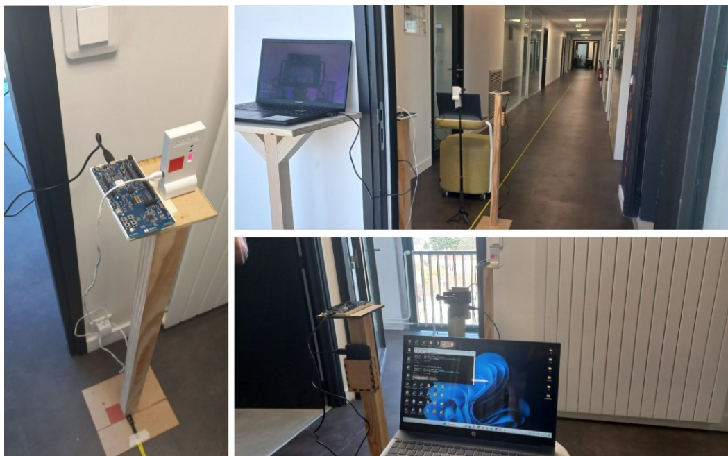
Figure 30: Forth floor's corridor of building A in the Villejuif campus will be obtained to conduct the interference test.
