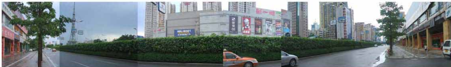
C 基地周边情况 Site Surrounding Areas
