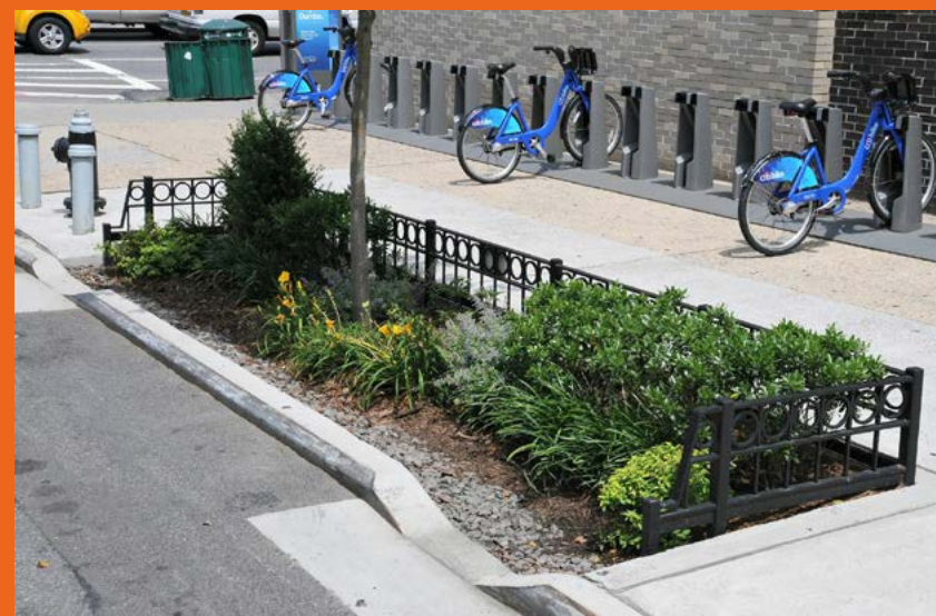
Bioswale lungo strada a New York. Fonte: NYC Department of Environmental Protection, in Schulz (2014)
