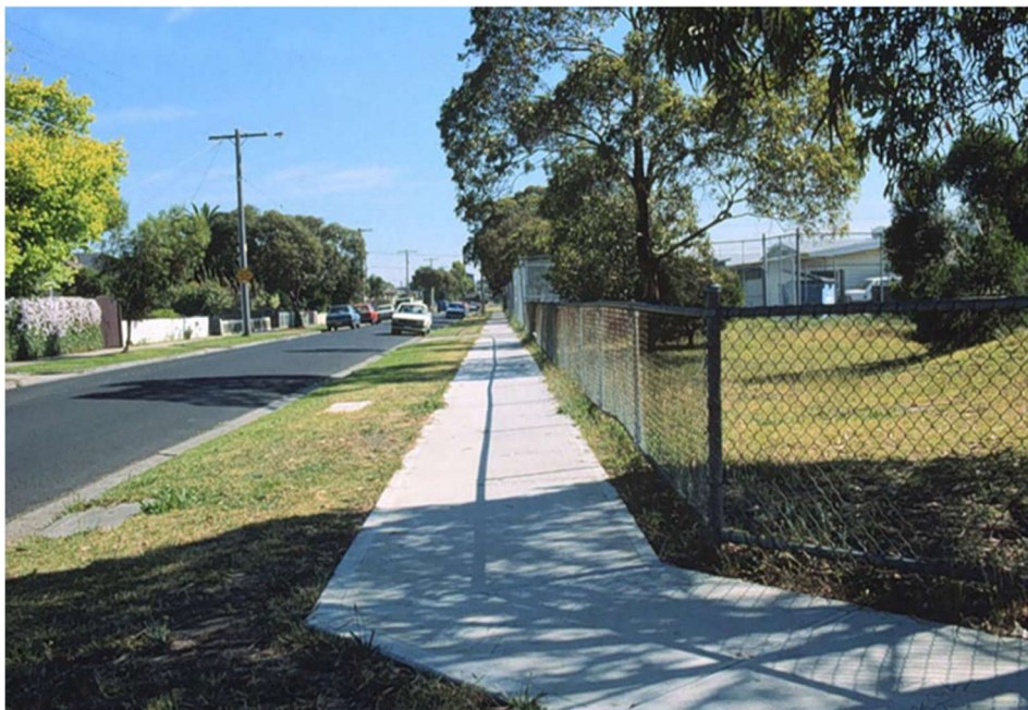
Figure 5. The footpath of Werribee south,Victoria .(Sagoe-Crentsil, 2002)
