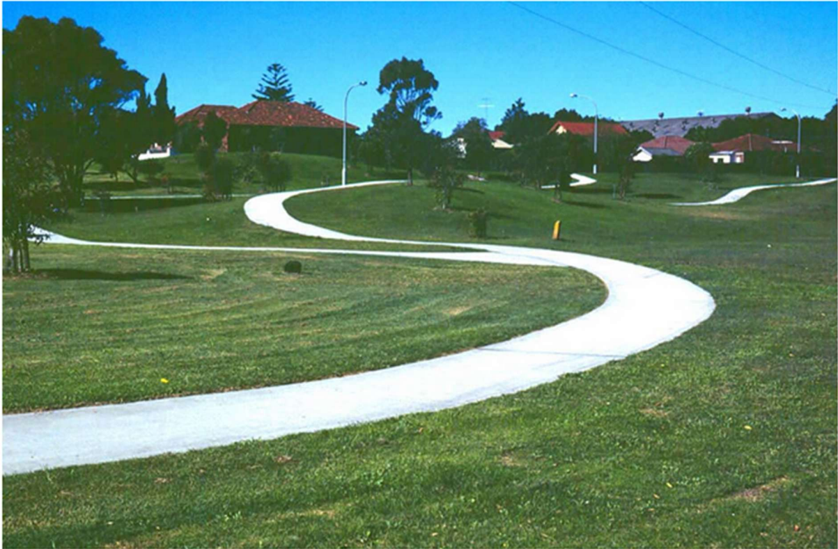
Figure 6. The footpath of Randwick, NSW constructed with 80% recycled aggregates.(Sagoe-Crentsil, 2002)
