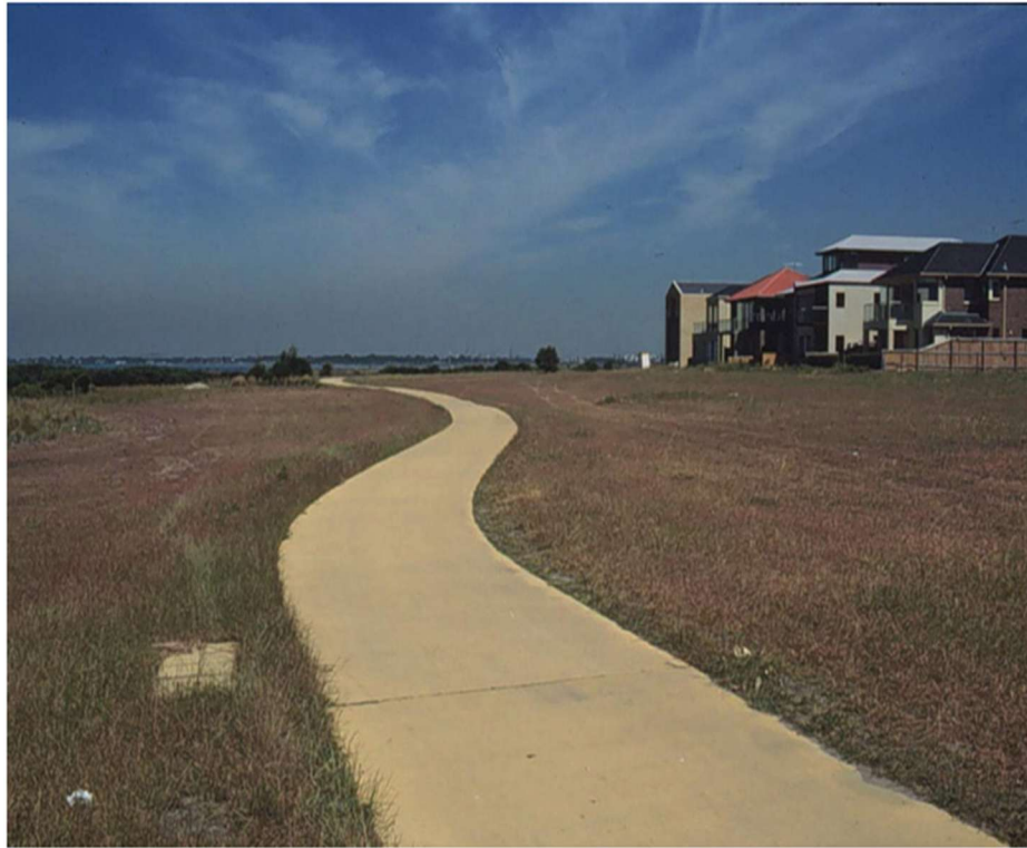
Figure 4. The walking/bike path of Williamstown,Victoria , using concrete incorporating 100% recycled coarse aggregates. (Sagoe-Crentsil, 2002)
