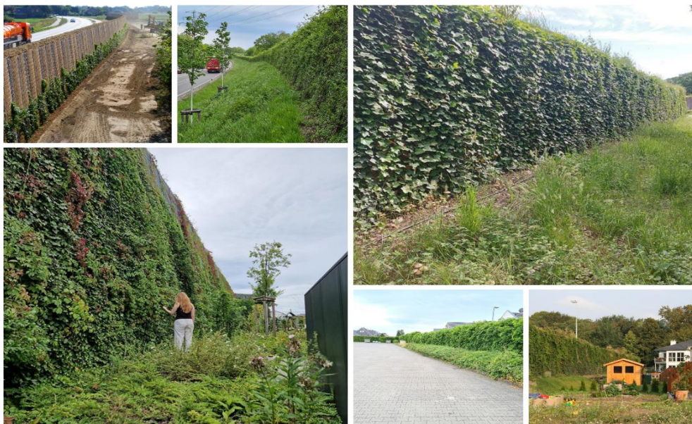
Fig. 13: Green noise barriers bring a piece of nature back into the city. Thanks to the innovative integrated trellis system of the Noise Guard Green, it is possible to green the noise barrier. Graffiti and other defacement on the noise barrier are concealed by climbing plants after a short time and are therefore virtually invisible to the observer.
