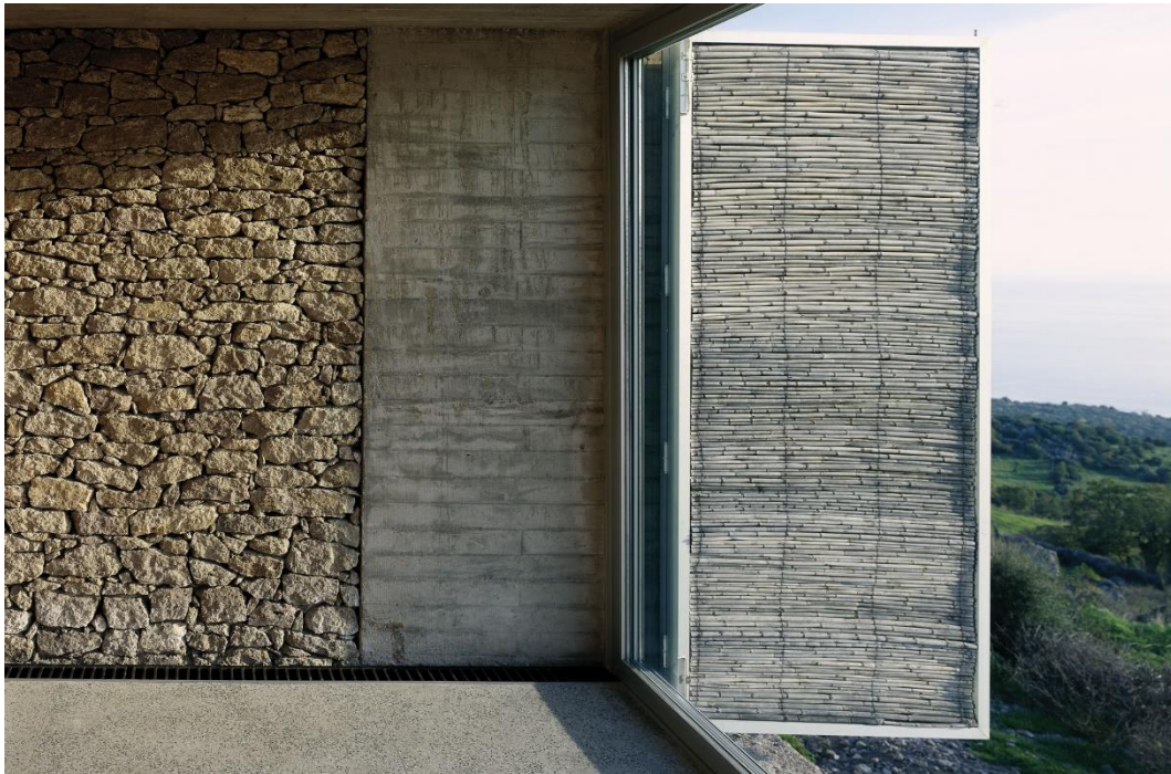
Figure 40. Raw Concrete and Handcrafted Stone Facade, Han Tumertekin, 2001, source: Aga Khan Trust for Culture.
