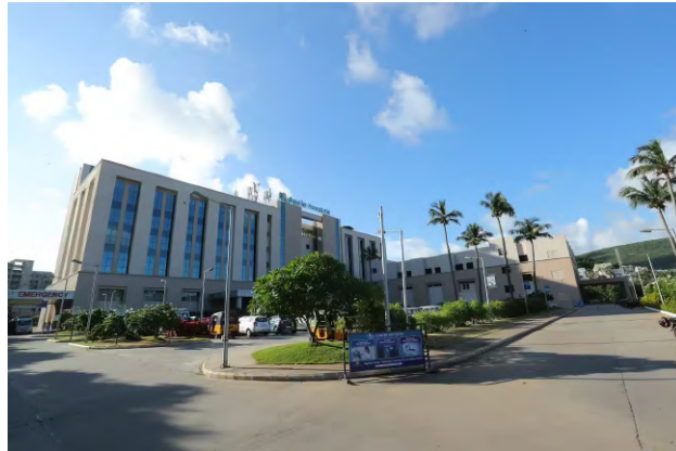
Figure 9.4: external view of one of the Apollo hospitals in Visakhapatnam.
