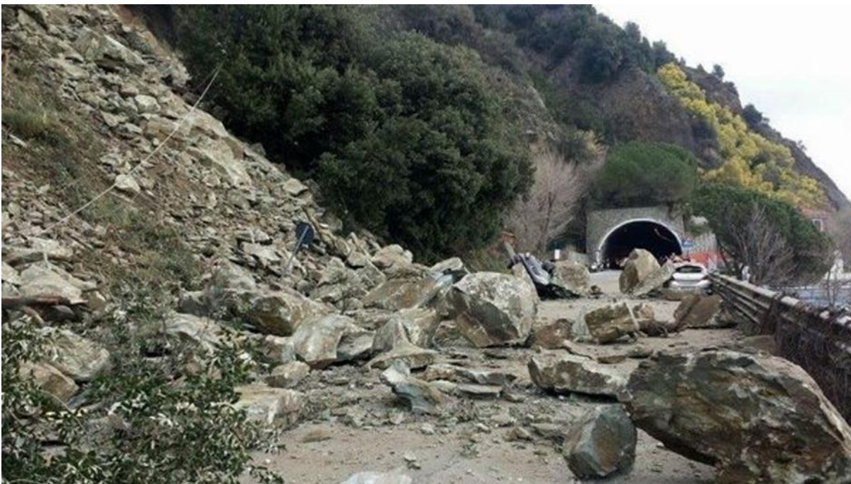
Figure 1. Landslide on the Aurelia road between Vesima and Arenzano (Genoa area) in 202c (source: https://www.today.it/citta/liguria-frana-aurelia-arenzano.html )
