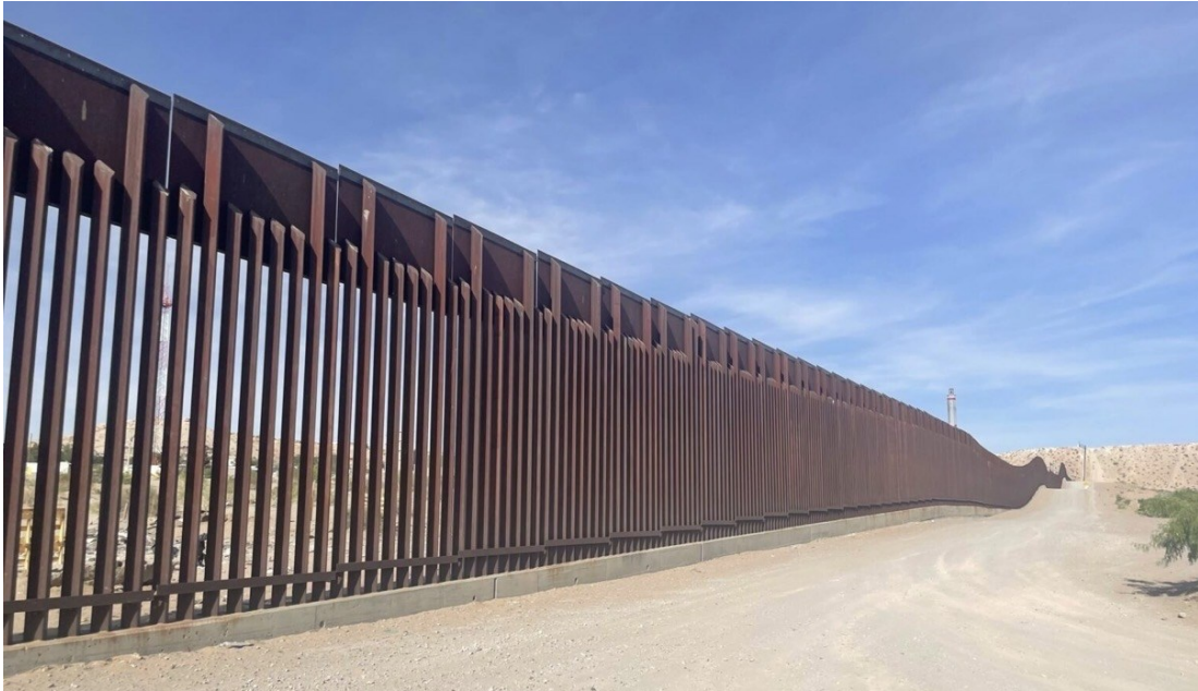
Figure 8 – U.S.–Mexico border wall near El Paso, Texas (2024). Example of contemporary steel bollard fencing used in recent phases of U.S. border fortification. Source: Ariana Figueroa / States Newsroom.
