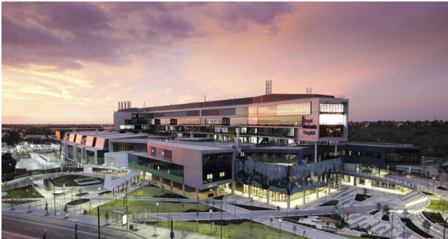
Figura 3 Royal Adelaide Hospital, Australia
