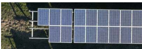
Figure 5.11: Incomplete panel line ending.
